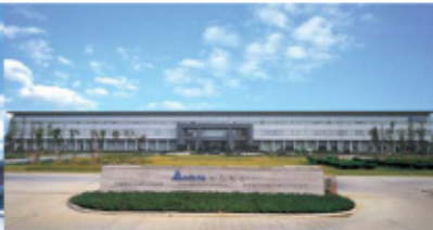
Manufacturing Plant in Wujiang, China
